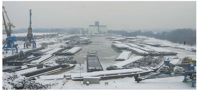
Berthing front - 720 meters. There are reloading facilities: portal cranes - 4/8 - 27.5, floating cranes - 1/5. Warehouse area: covered - 32,000 sq.m., open - 180,000 sq.m. There is also a rail connection.
