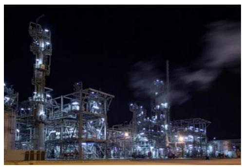
The refinery's production facilities are located on over 500,000 square meters in the Salina district of Alexandria and consist of two complexes: a lubricating and specialty oil complex, which produces neutral oils, solid paraffin, soft paraffin, and aromatic oils, and a gasoil facility. a complex producing gasoil, naphtha, and LPG for local
