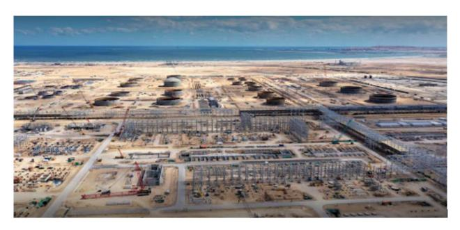
The facility will use a total of eight crude oil storage tanks with a capacity of 550,000 barrels each at Ras Markaz. An 80.7 km long, 28-inch diameter underground pipeline will be constructed to export blended crude oil from the Ras Markaz crude storage tanks to the Duqm refinery.
