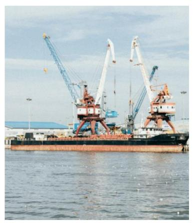
The mooring front is 800 meters, whereas the mooring front is 100 meters, and the sloping coast is 700 meters. There are handling facilities: portal cranes - 6/5 - 20, floating cranes - 2 / up to 6. Warehouse area: covered - 21,000 sq.m., open - 600,000 sq.m. There is also a rail connection.
